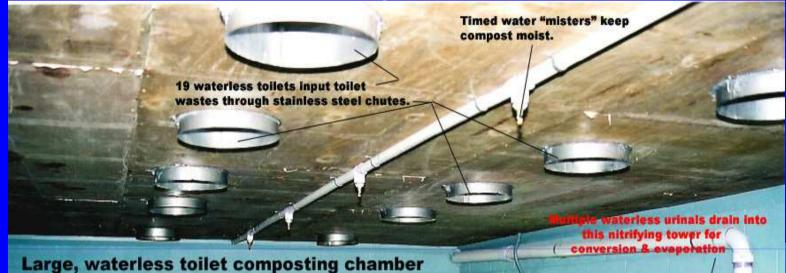
Receives 350,000 toilet uses in 5 months. No flush water, no sewage, no odor, no chemicals, no pump-outs. Saves 1,000,000 gallons of fresh water and prevents over 1,000,000 gallons of sewage from discharging to the environment per season.
